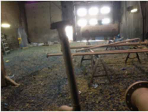
Spools & Vessel sandblasted
